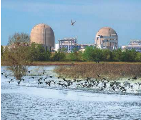
South Texas Project Electric Generating Station
